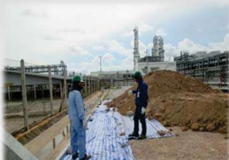
Prevent soil falling to drainage
